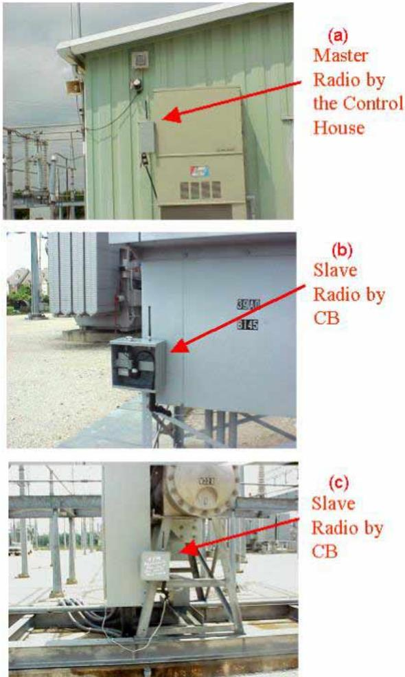
Fig. 1. Equipment disposition
